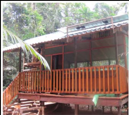
Luxury accommodation including solar power added to the Eco-tourism offering
